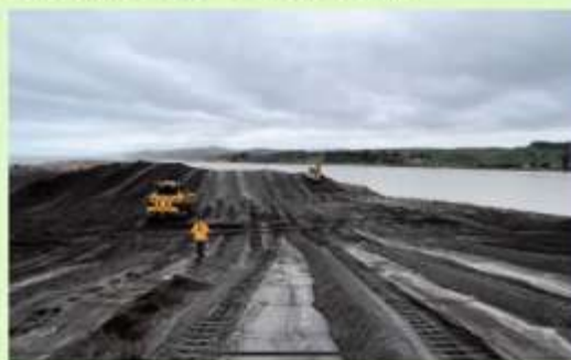
Overflow channel being created in the Wairoa Bar, east of Pilot Hill and adjacent to the old training structures
