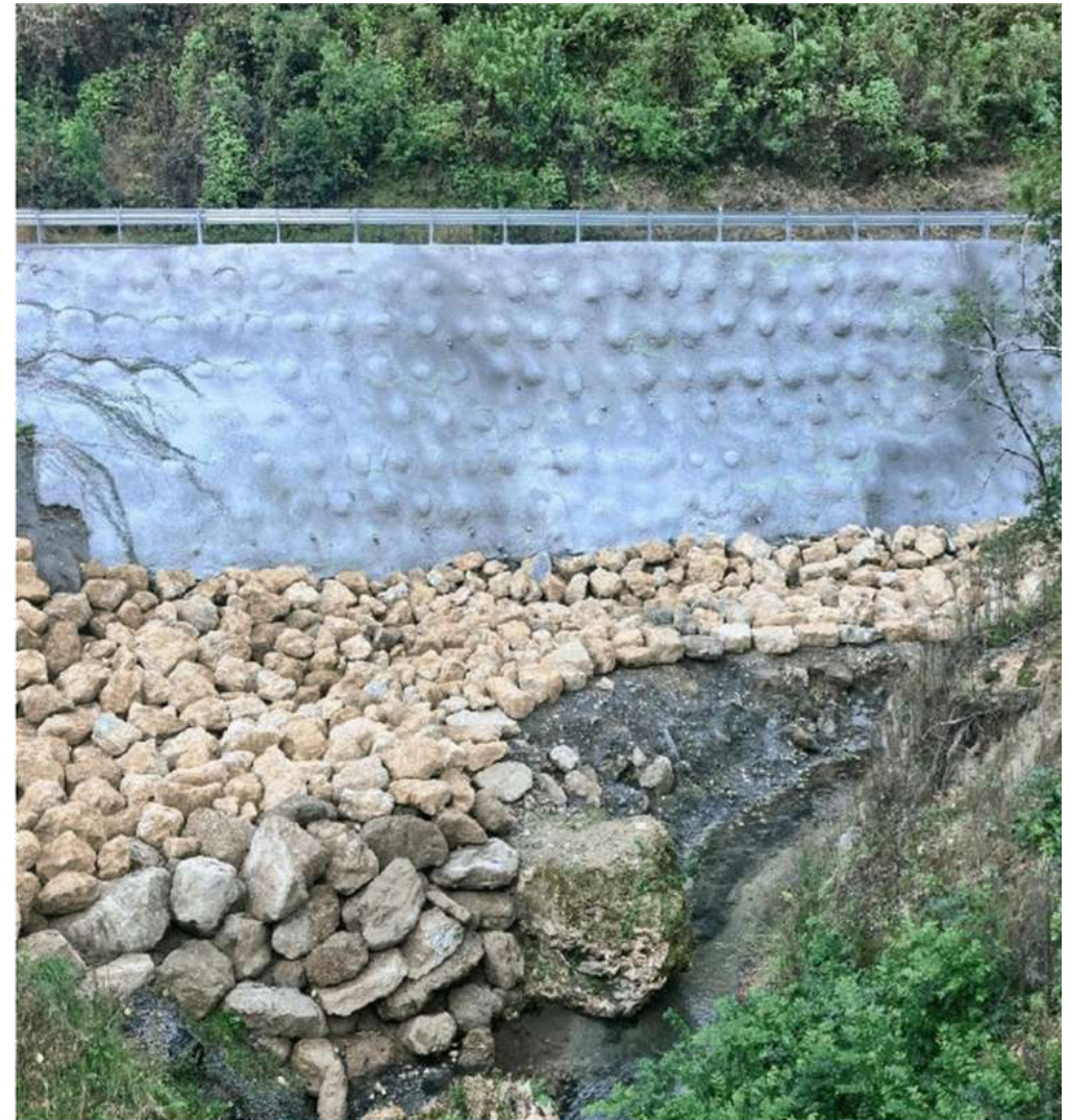
White Pine Bush wall – riprap working well, no scouring
