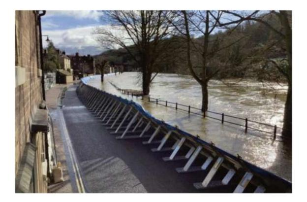
Option 14 involves creating street-level flood protection through the installation of structures to protect houses and buildings. *Example shown above.*
