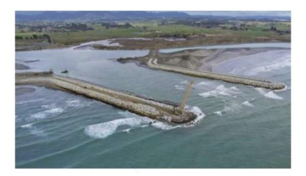
Option 12 involves creating a permanently open river mouth by creating engineered structures. This option does not prevent flooding in North Clyde.
