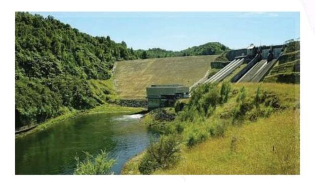
Option 9 involves building a series of small dams in the upstream catchments, or large in-river dams, to store water and try to slow the peak rate of water flowing into the Wairoa River. Above is an example of the Patea Dam in Taranaki.
