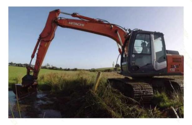
Option 15 involves clearing out and maintaining the existing drainage network throughout North Clyde, creating more drains or enlarging existing drains to accommodate more water volume, and/or clearing out the Awatere Stream and increasing its width to increase flood carrying capacity. This option would not prevent the flooding of North Clyde from the Wairoa River.
