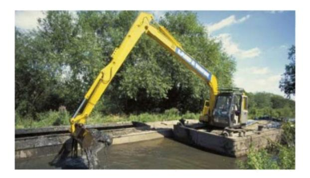
Option 11 involves dredging the Wairoa River channel to increase the river's flood carrying capacity. This option would require an extremely high quantity of material to be removed from the river for any notable flood reduction benefit for North Clyde.
