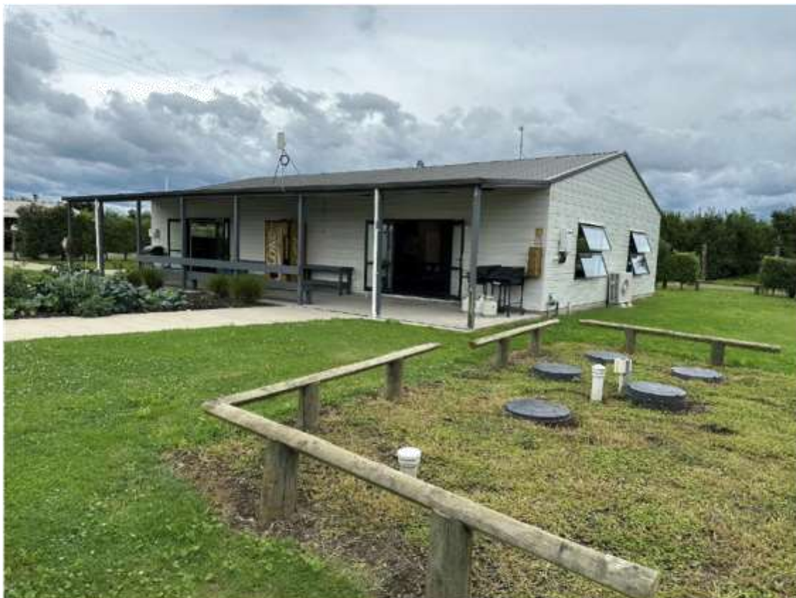
Image 8. A typical multi-chamber domestic wastewater treatment system
