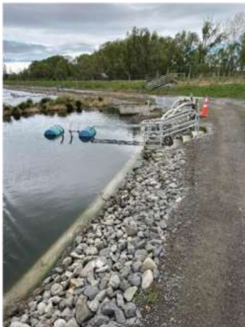
Image 10. Wastewater treatment pond at Waipukurau
