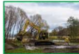
Site establishment for Puketapu Bridge, 17 June 2024
