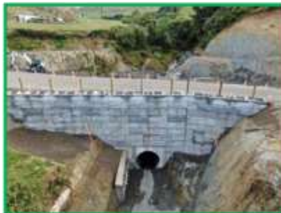
Chrystal Culvert nearing completion, May 2024
