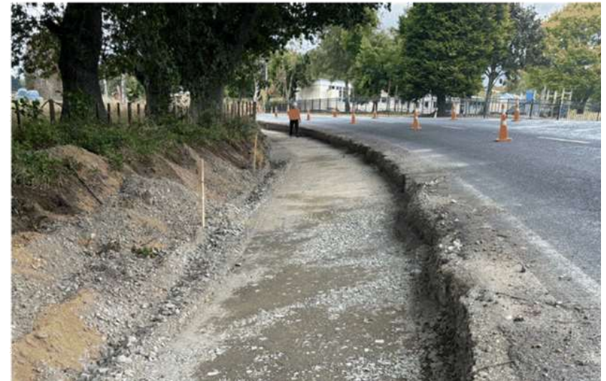
Work in progress at Kakariki (bottom)
