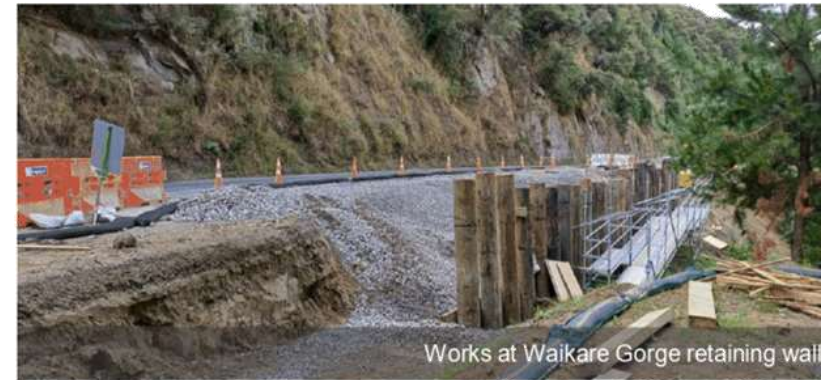
Building the retaining wall at Devil's Elbow
