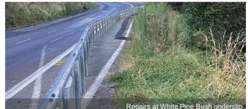
Repairs at White Pine Bush underslip
