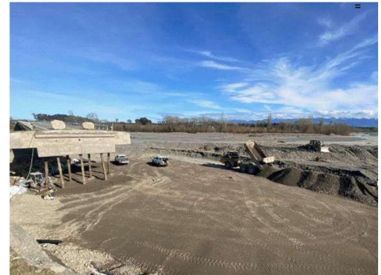
Waipawa River Bridge repairs – 20 July (bottom)
