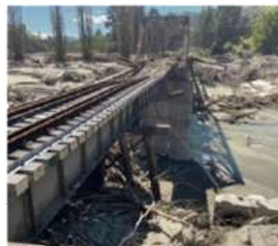
Damage to a bridge in Esk Valley
