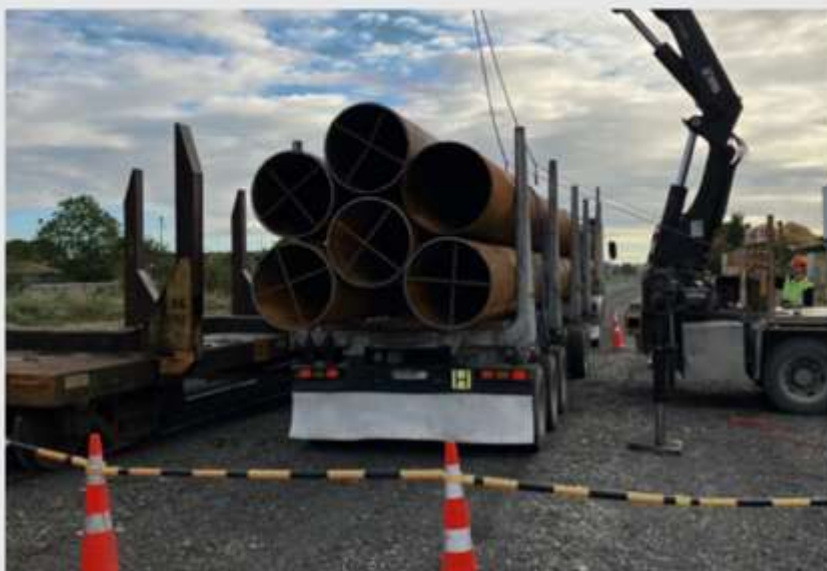
Steel pile casings being loaded onto a rail carriage in Christchurch for Napier bridge repair
