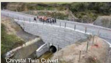
Chrystal Twin Culvert
