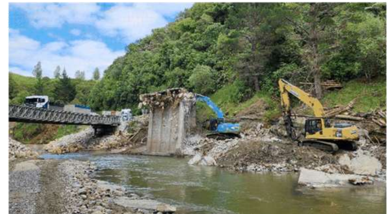
Cyclone-damaged Waikare Gorge bridge being demolished late 2023. (Bailey bridge installed mid 2023).
