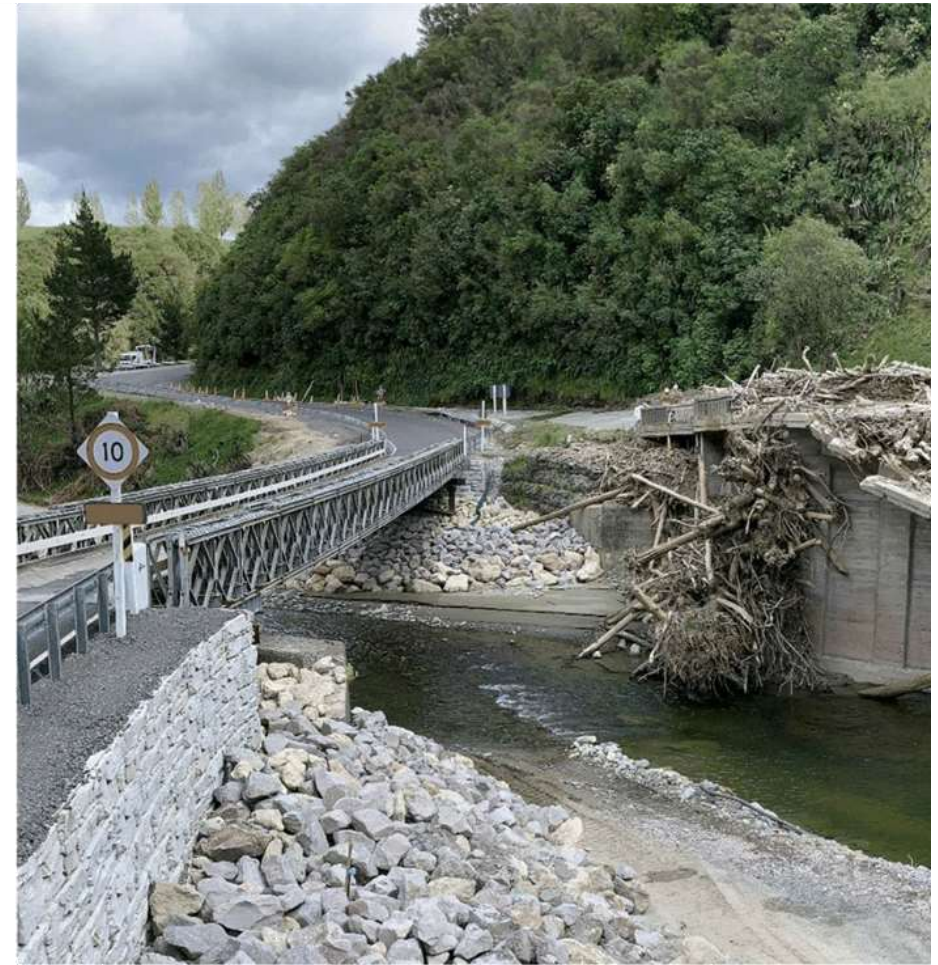
Bailey bridge over Waikare Gorge and prior to demolition of Cyclone damaged bridge.
