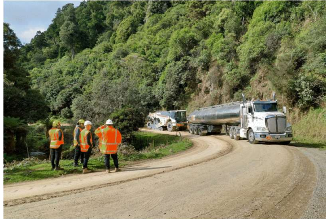
Inspection of tall oil pitch application
