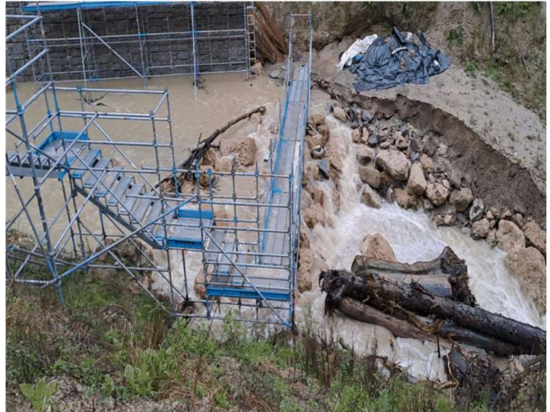
Late June weather event: rock scour at Devil's Elbow did its job well, mass block remained in place.
