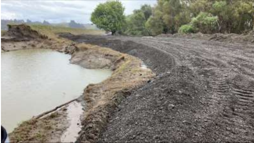
Figure 1: Temporary bund in Waipawa
