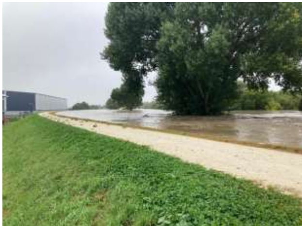
Figure 4: Taradale stopbank holds
