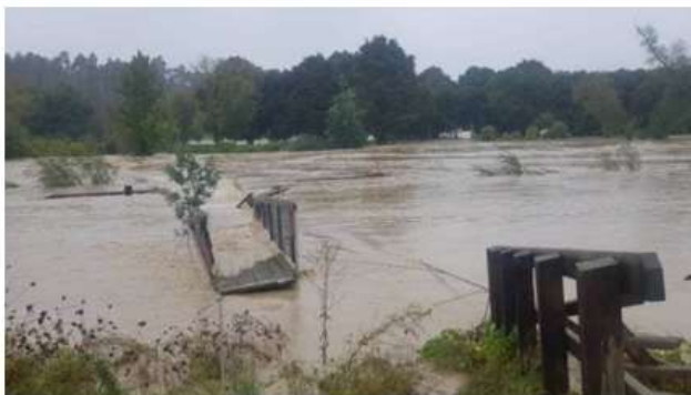
Damaged Upper Tukituki Cycleway Tarewa Swing Bridge
