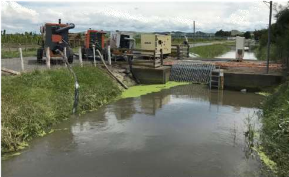
Figure 37 Mobile pumps and generator at Waverly pump station
