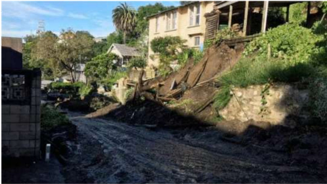
Figure 87: Roading damage on Brewster Rd, Napier Hill.
