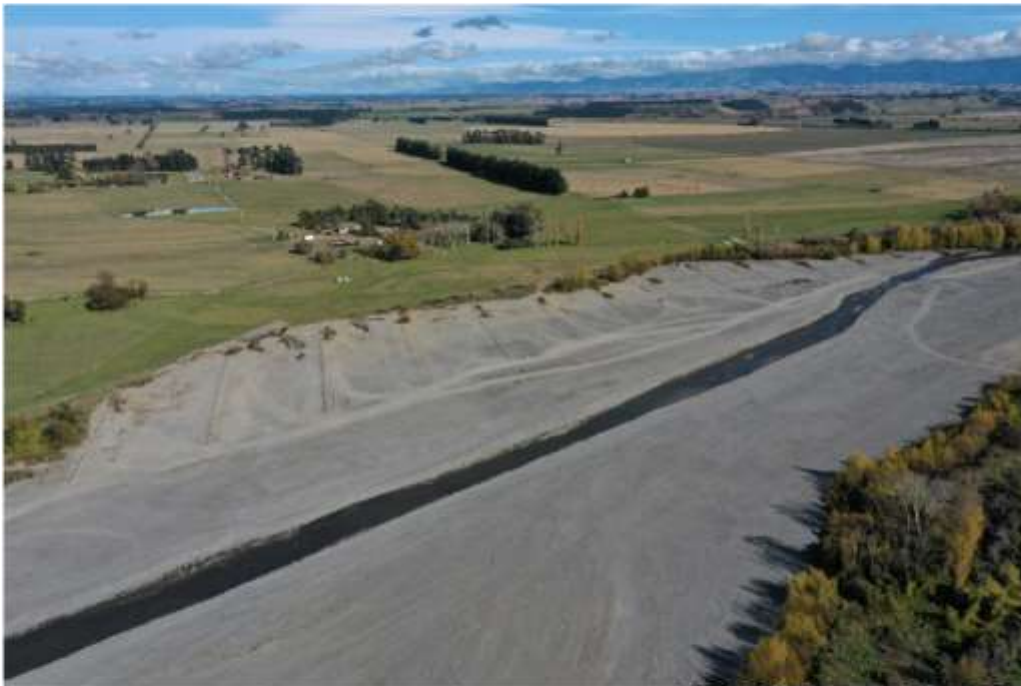
Figure 2 SH-50 Waipawa River - Right bank permeable groynes near completion
