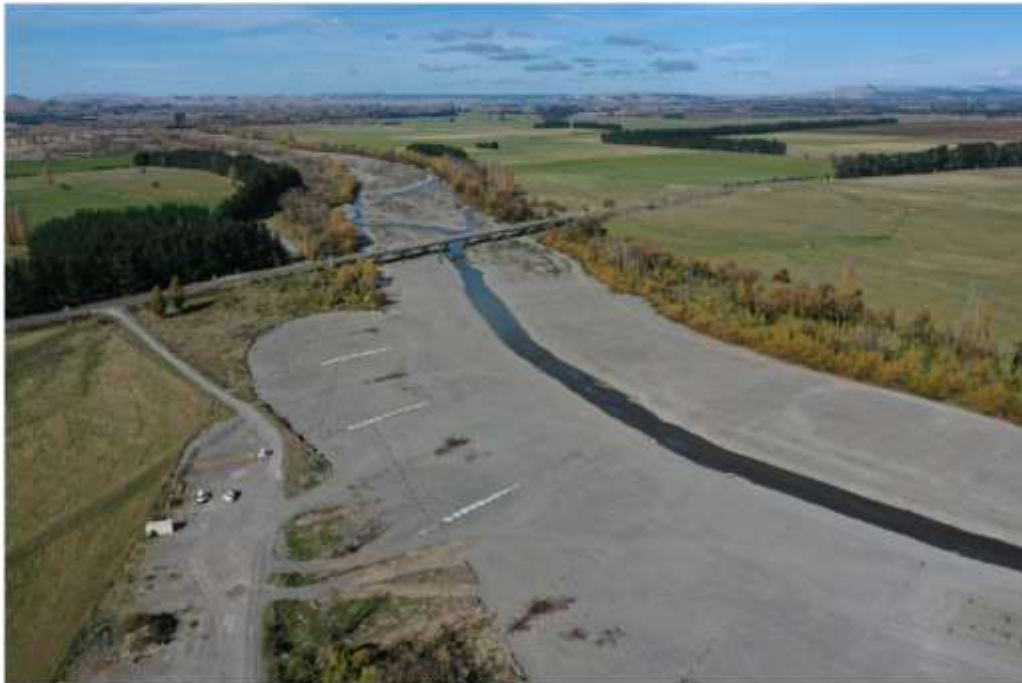
Figure 1 SH-50 Waipawa River - Left bank completion of permeable groynes, akmons and earthworks
