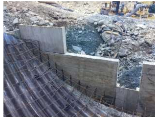
Steel tied into new abutment wall at inlet.
