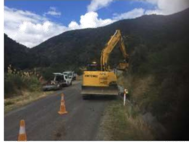
Set up De-watering Pumps and diversion pipes
