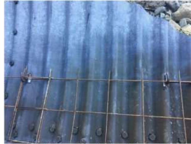
Stream diverted, culvert base cleaned and working platform constructed to allow welding of hooks to support Reinforcing mesh.
