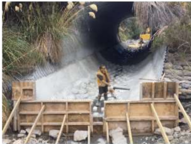
Cleaning off to apply curing compound
