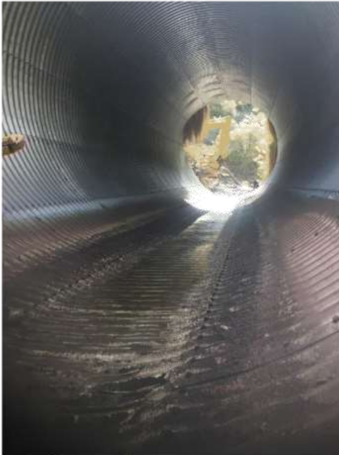
Extensive corrosion in base of culvert
