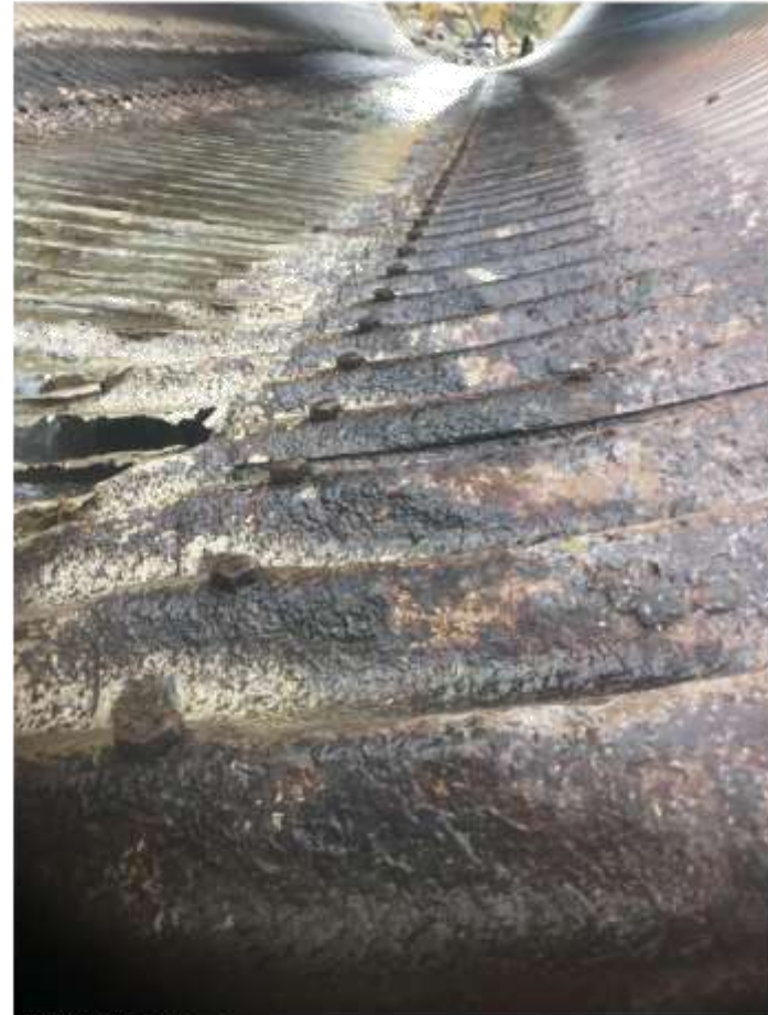
Extensive corrosion in base of culvert
