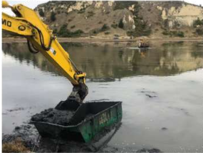
Unloading the skip bin directly into truck
