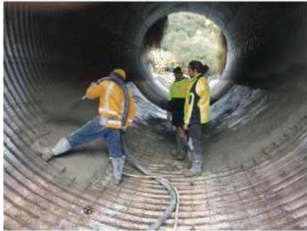
Shotcrete 40Mpa Fibre reinforced concrete
