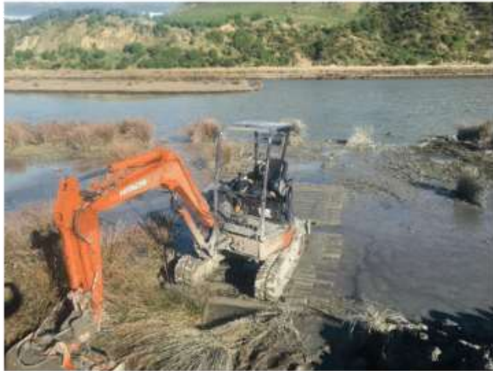
3 Tonne digger on swamp pads
