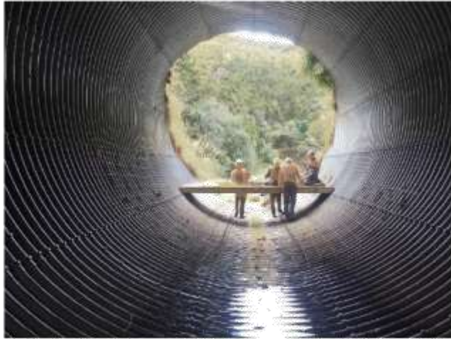
Stream diverted, culvert base cleaned and working platform constructed to allow welding of hooks to support Reinforcing mesh.
