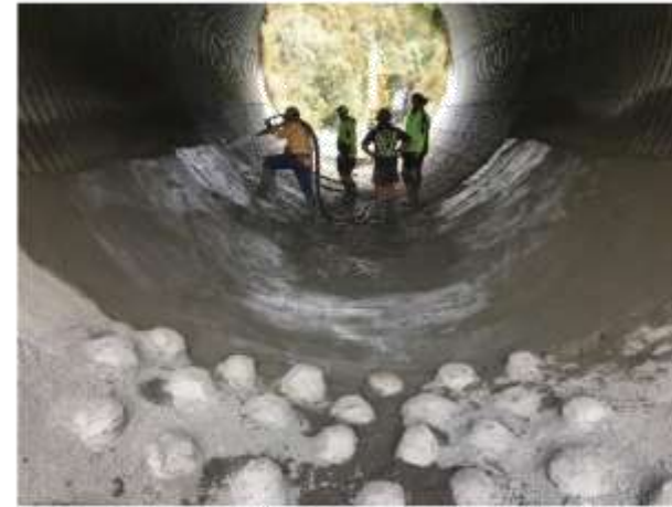
Fish refuge formed as one with the slab using concrete
