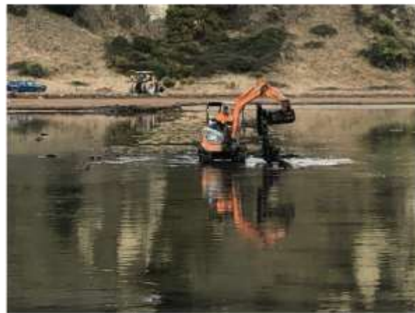
Shifting the swamps pads into position
