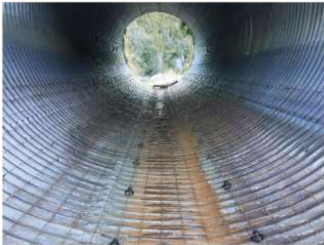
SE72 reinforcing mesh welded to culvert
