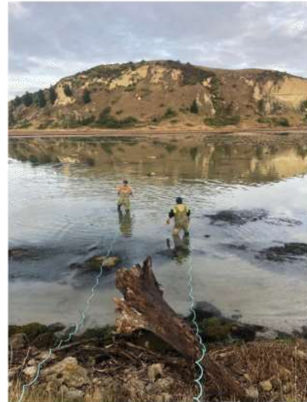
Setting draw line for the 500m steel cable
