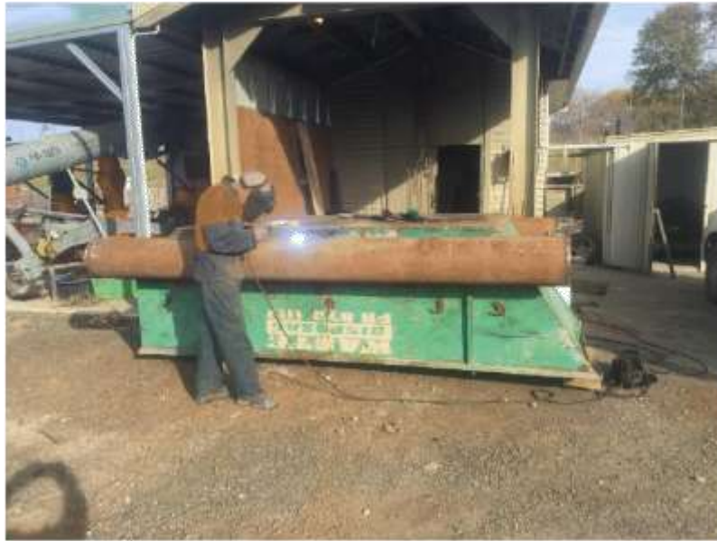
Welding pontoons to the skip bin
