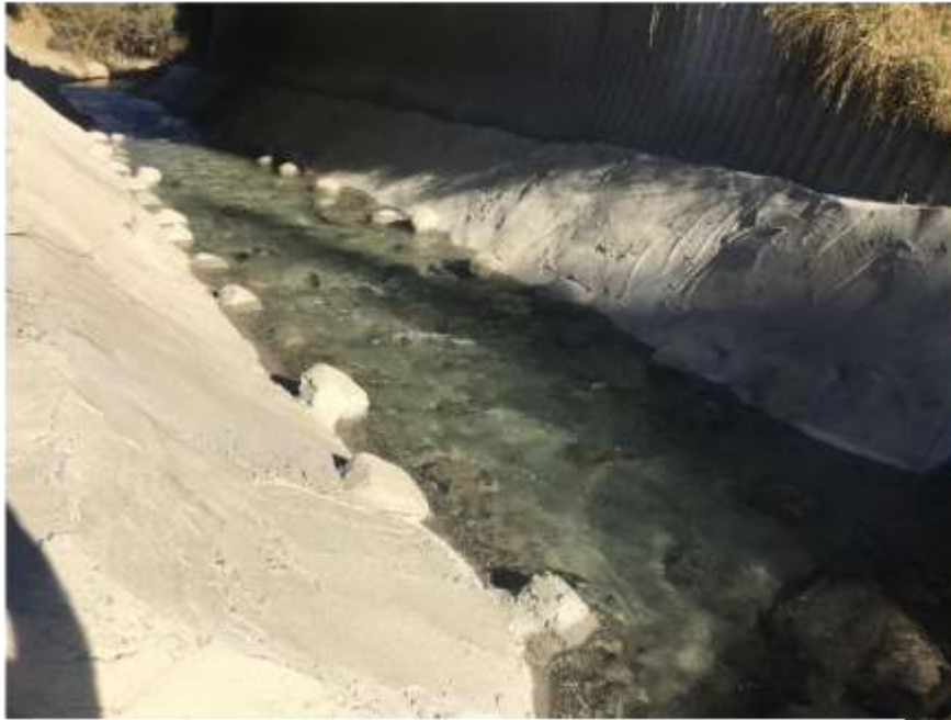
Water released after three days of curing
