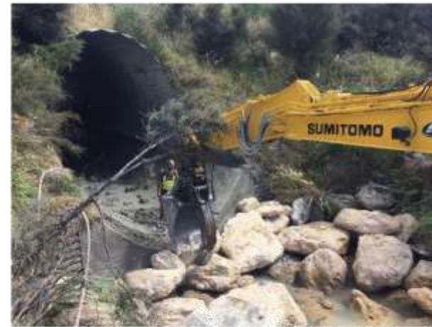
Placing lime rock at outlet before shotcrete
