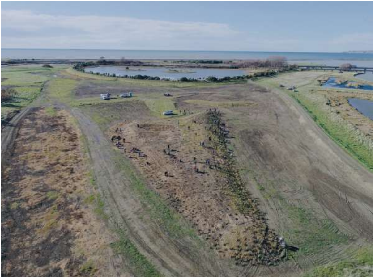
Fig. 7: Drone image of the volunteer planting of the largest of 3 islands.
